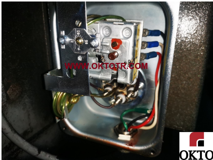
WRONG ADJUSTED HEATER OR DEFECTIVE THERMO VALVE
